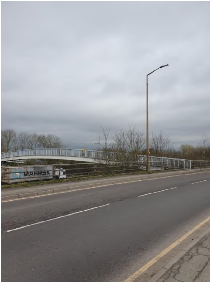
Photo 2.4: London Road looking towards the footbridge over the A12
