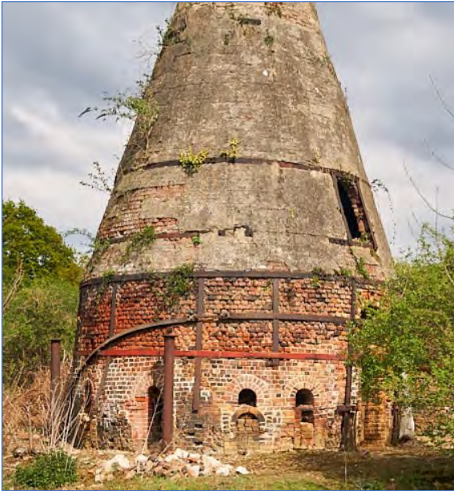
Figure 4 The western circular brick kiln, scheduled and Grade II listed © WH Collier website
