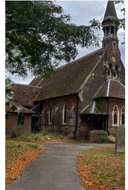
Figure 16 St John's Church is a Grade II listed building neighbouring the site
