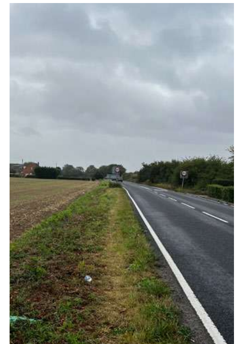
Figure 19 Absence of pedestrian infrastructure extending along Harwich Road
